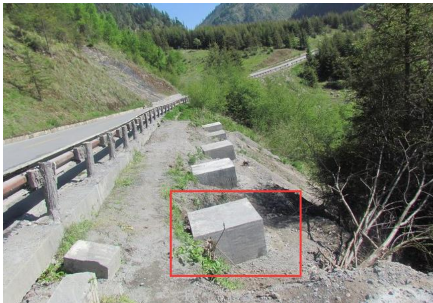
Anti-slide piles (all below the terrain)
